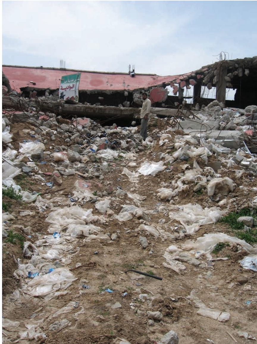
Bulldozer tracks are visible leading to the remains of the Al Wadiyya family's destroyed biscuit factory, in an industrial area near Izbt Abd Rabbo. © 2009 Bill Van Esveld/Human Rights Watch.
