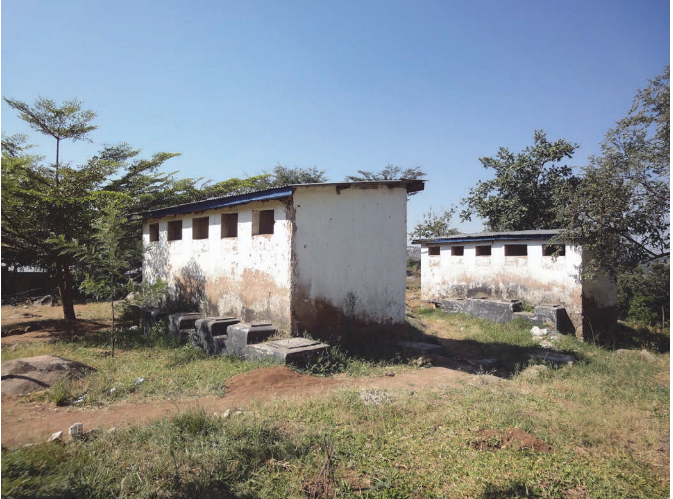
Female and male latrines at a secondary school in Mwanza, northeastern Tanzania. Many students told Human Rights Watch that they had to use dirty and congested pit latrines. © 2016 Elin Martínez/Human Rights Watch
