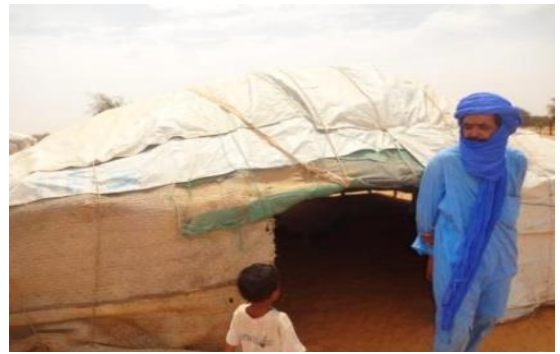
Example of a traditional shelter to be restored for refugee returnees in the commune of Gossi in the region of Timbuktu, credit ©UNHCR Gao
