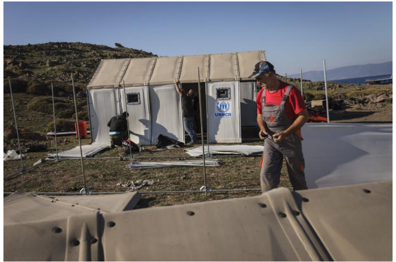
Refugee Housing Units are being set up along the beaches of Molyvos, Lesvos ©UNHCR/A. Zavallis
