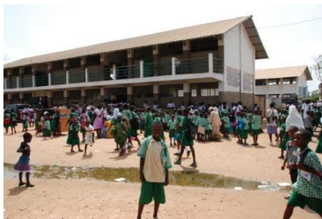
Fig. 38: School built through FIOH's Construction and Technical Programme (© Future in Our Hands website)
