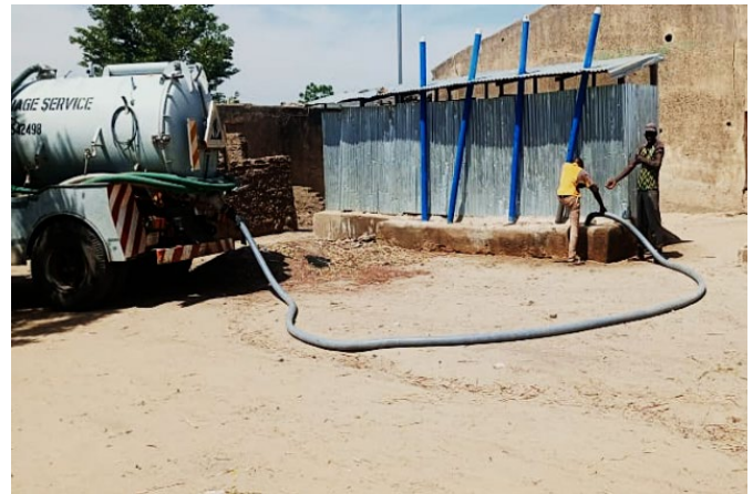
Desludging filled latrines in Dikwa, Borno State Photo: Norwegian Church Aid
