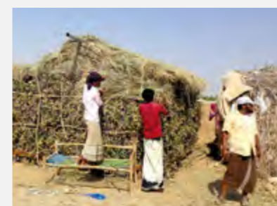
Internally displaced Yemenis construct their own eco shelters using natural materials near the town of Abs in the north-west of the country.
