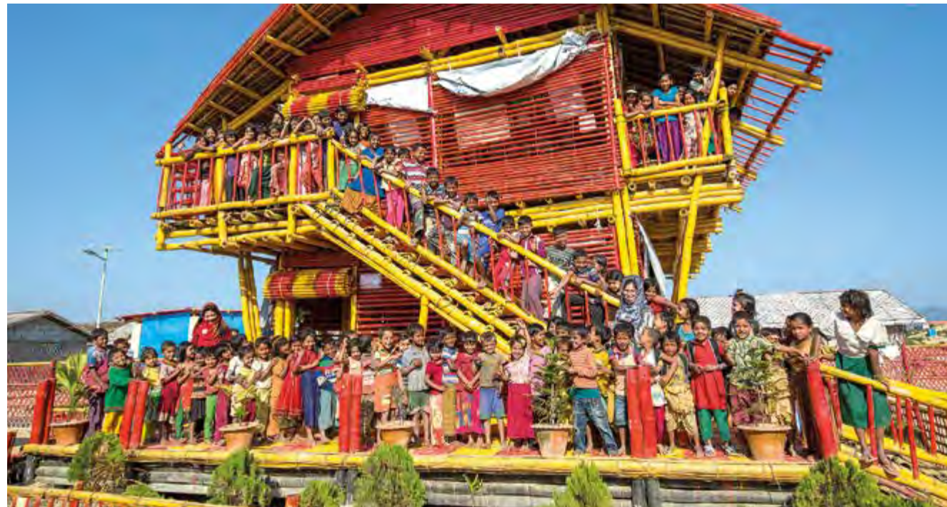
Sunflower Learning Centre in Kutupalong Extension Camp 4, Bangladesh, is the first two-storey building in the camp and was designed to save space and reduce overcrowding.
