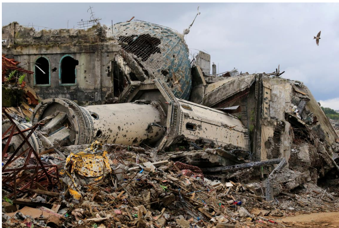
Damaged houses and a mosque are seen in Marawi city, 25 October 2017. © Romeo Ranoco/Reuters
