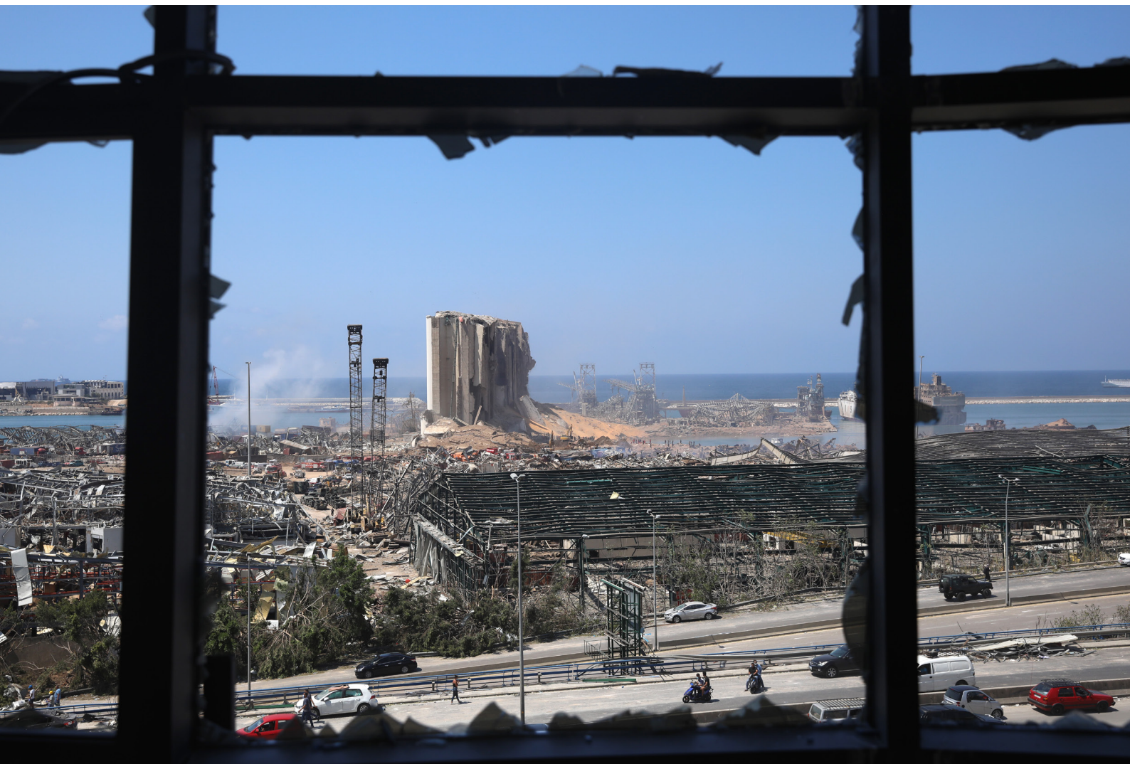
The ruins of the giant grain silos stand amid the devastated port of Beirut. Photo: ©UNHCR/Houssam Hariri
