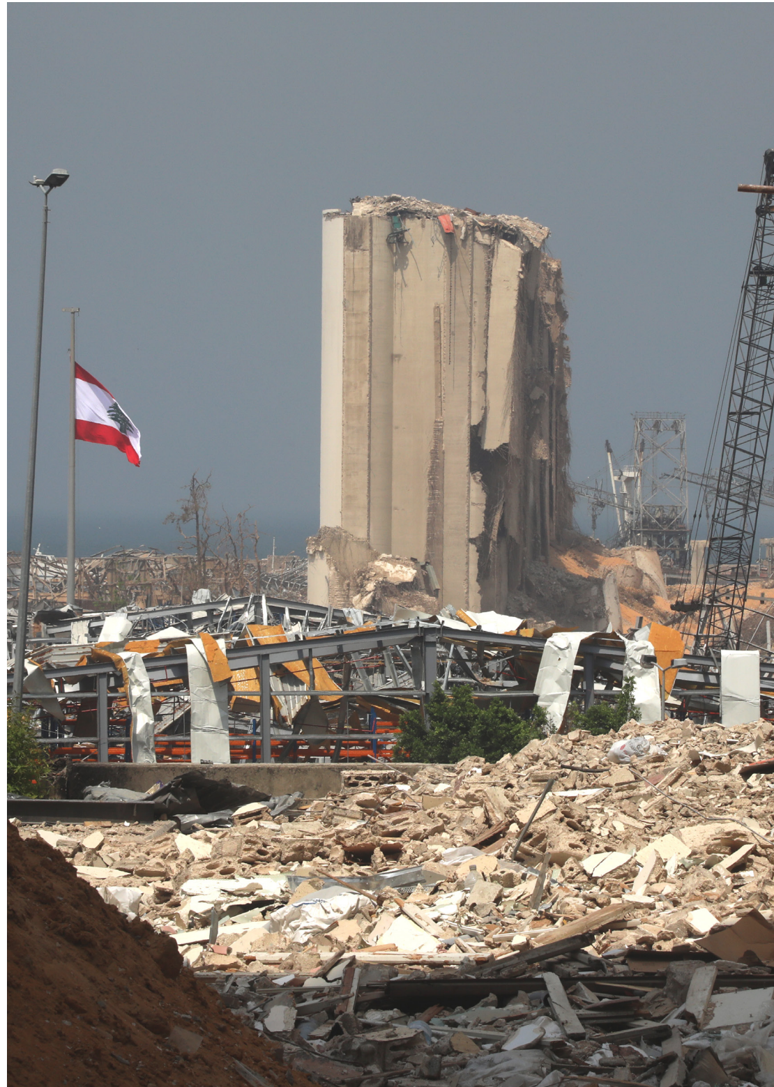
The devastation caused by the Beirut port explosion. Photo © UNHCR/Houssam Hariri
