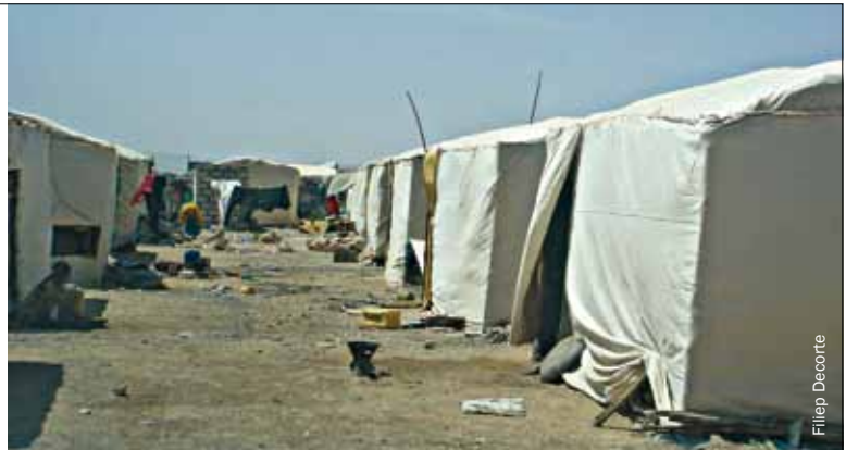
Upgraded IDP settlement with fire breaks, Bossaso.
