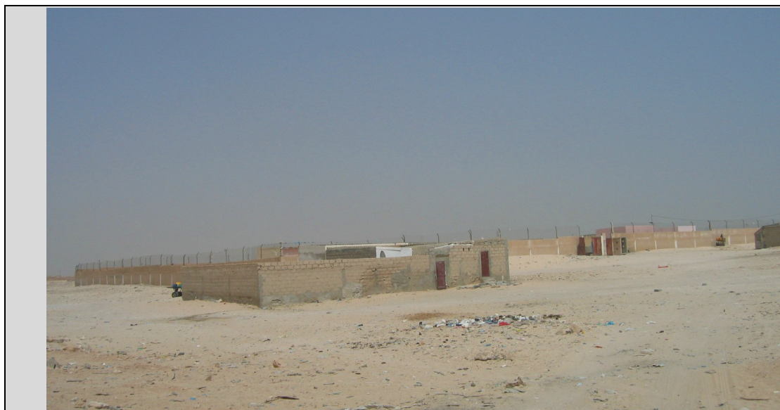
© AI – Nouadhibou Detention Centre
