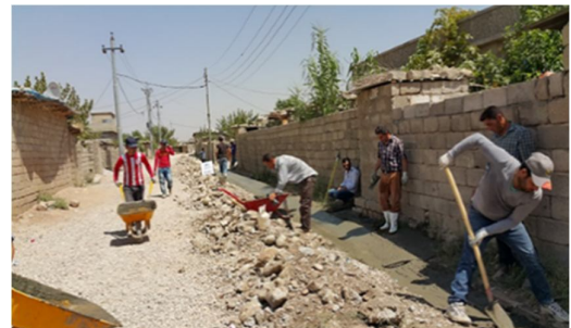
Construction of open channels in Husseiniya Settlement (UNHCR/H. Fahmi)
