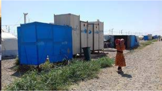
Latrines in Hamam Al Alil 2 camp
