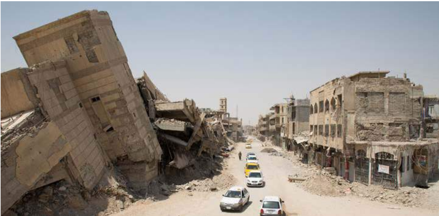
A view of Mosul's Old City. Photo: NRC/Tom Peyre-Costa, July 2018
