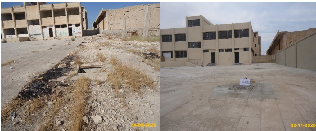
Rehabilitation of the vocational school in Souran, Hama © SIF.
