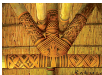
Coconut fibre tying for roof trusses (left) and corner post-ring beam (right)
