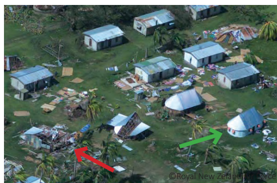
Cl sheet bure after cyclone Winston: even if some have been damaged, they have resisted better than other constructions
