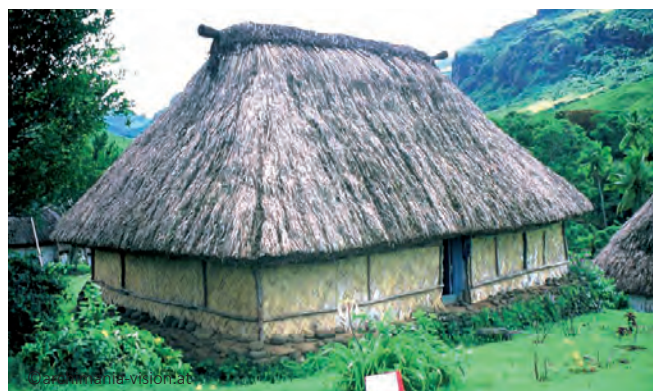
Traditional house: woven mat walls are fixed on the outside with additional wood elements to improve resistance to wind pressure; the top of the roof is reinforced with an additional layer of special grass tied to a timber beam protruding from two sides of the roof
