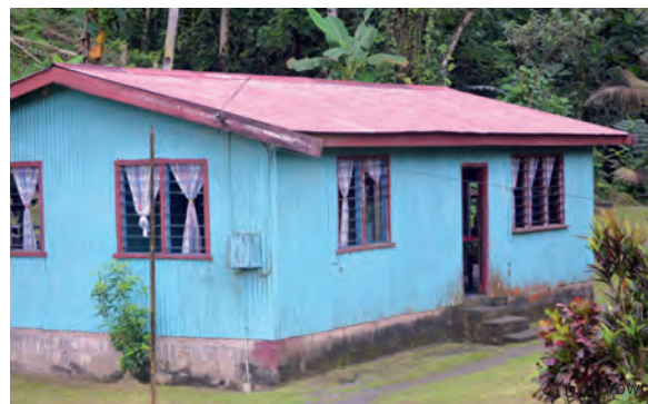
Formal timber-framed house on cement block plinth
