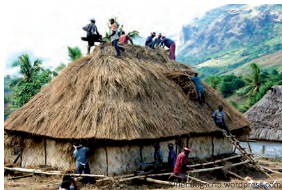
Housing construction with the involved of the community
