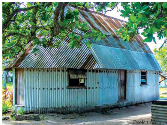
Bure built using Cl sheets as evolution of the traditional building practices: round shape for improved aerodynamicism
