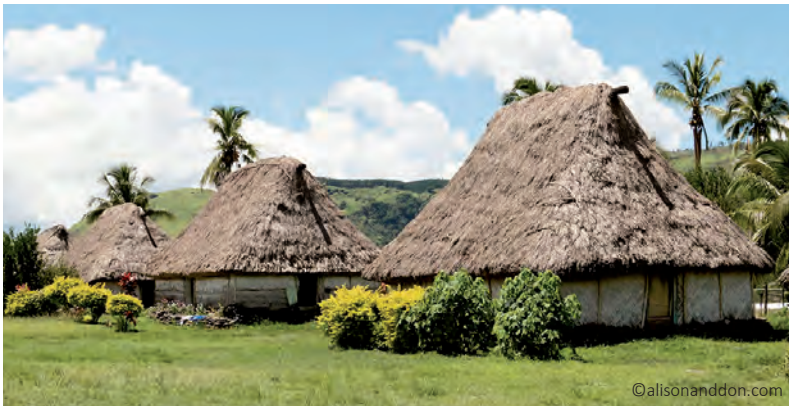
Traditional housing: lightweight flexible construction and 4-slope hipped roof for better wind resistance
