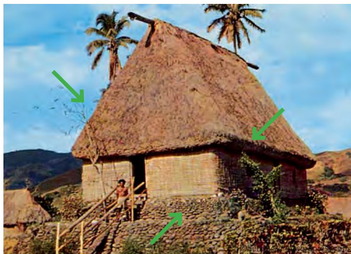
Elevated stone platform for protection from floods and soil erosion. Small eaves and steep roof for reduced vulnerability and improved durability
