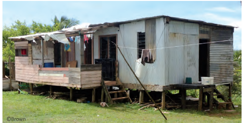
Transitional CI sheet housing: elevation on stilts for better protection from floods
