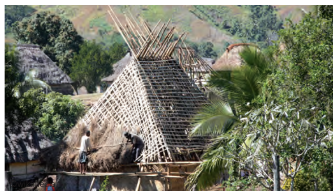
A net of woven reeds is applied on the rafters to better fix the thatching
