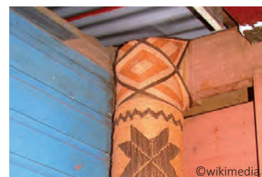
Coconut fibre tying for roof trusses (left) and corner post-ring beam (right)
