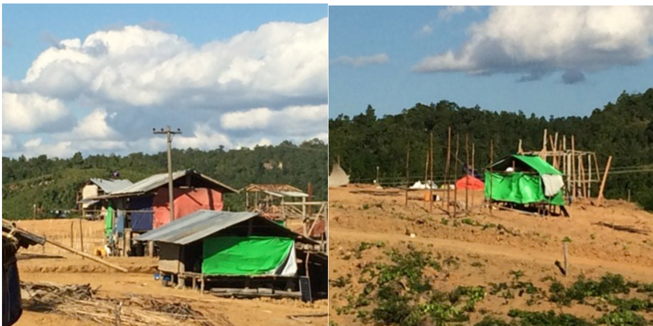
Self-reconstruction on Mowlaik relocation site (SCT, 27/11/2015)
