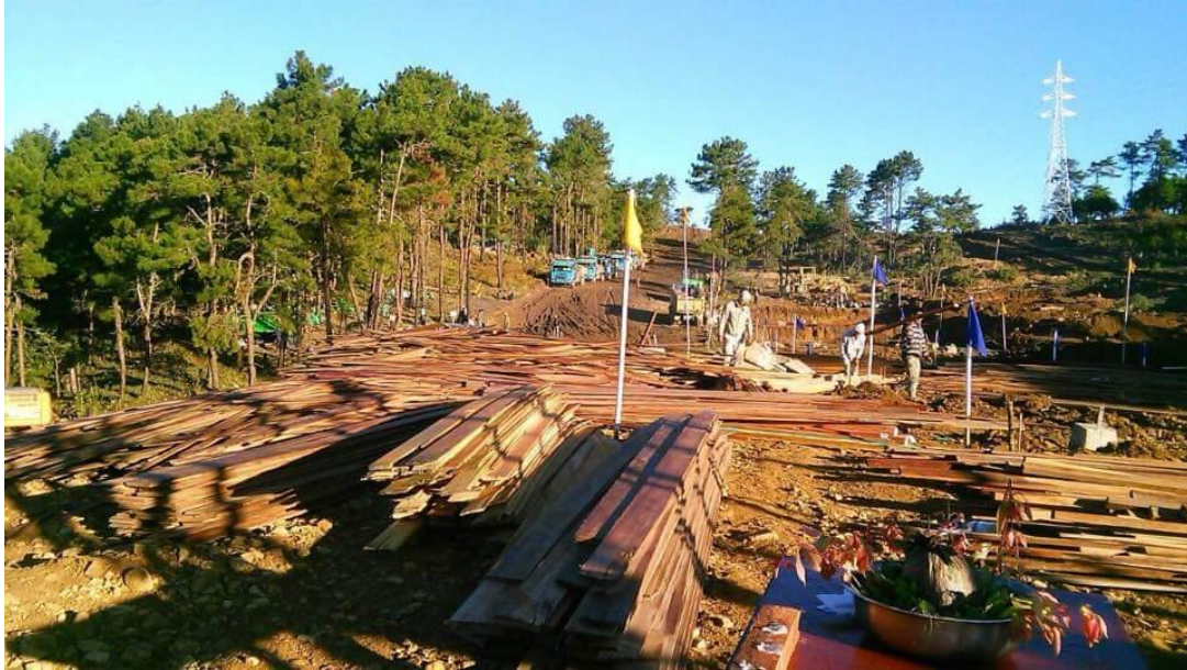
Relocation site in Hakha: Phase 1 underway for 380 plots (Courtesy of CHRO/October 2015).
