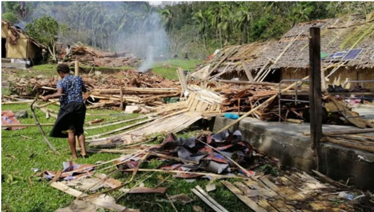
Vanuatu Business Resilience Council Damages after TC Harold 2020
