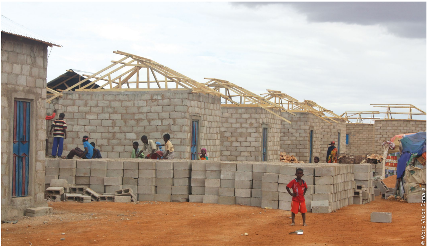
The project built 1,200 permanent houses with accompanying infrastructure across two new sites (here, the site in Garowe).
