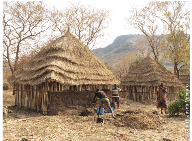
South Sudanese refugees in Tierkidi camp in Gambella, Ethiopia, plastering the walls of the shelters with mud sourced locally by themselves, in areas agreed with authorities and host communities.
