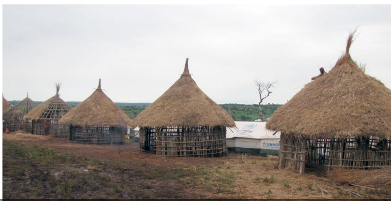
Timber and bamboo frames shelters were built with thatched roofs as a more durable shelter solution than tents. It proved challenging to source mud to plaster the walls as originally intended. Photos: Left: UNHCR, Right: Demissew Bizuwerk / IOM Ethiopia.
