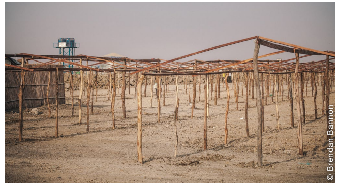
Shelter frames were built by contractors.
