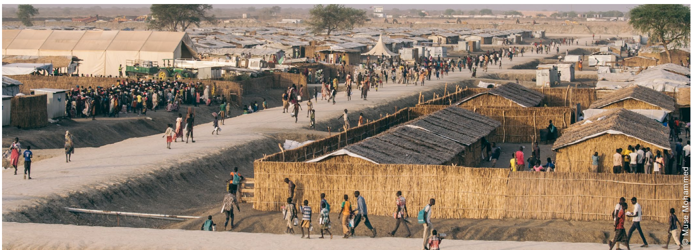
Bentiu Protection of Civilians site in South Sudan. This site for displaced people fleeing conflict has grown to over 120,000 people at its peak and has been upgraded over two years to improve living conditions, reduce health and safety hazards, and address the high increase in population.
