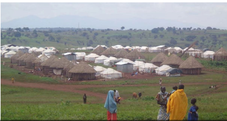
Timber and bamboo frames shelters were built with thatched roofs as a more durable shelter solution than tents. It proved challenging to source mud to plaster the walls as originally intended. Photos: Left: UNHCR, Right: Demissew Bizuwerk / IOM Ethiopia.
