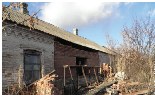
Interventions included housing repairs (Starohnativka, Dec 2015).
