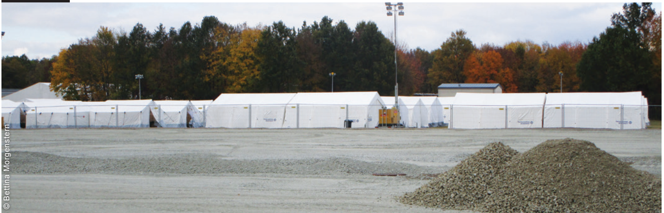
The reception centres were upgraded/winterized, while in operation, through several steps between October and December (e.g., by adding a layer of gravel).
