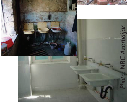
Bathrooms before and after upgrade
