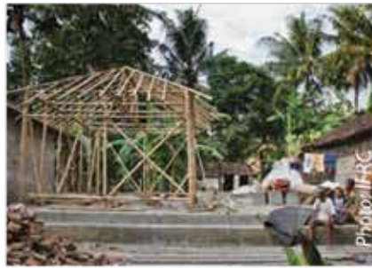
A transitional shelter built on the site of a destroyed house
