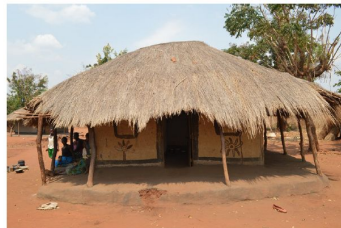
Verandas and large roof overhangs between the interior earth wall and the exterior avoid the risk that changes in humidity associated with rain will swell the soil under the walls. House in Simwaka, Nkhotakota. © Jon Twingi
