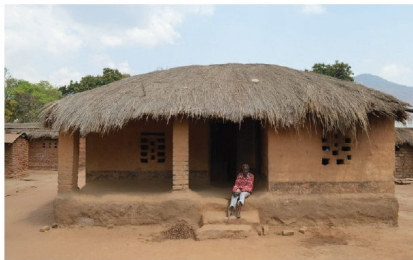
Houses constructed using adobe bricks, render and earth mortar like this one (Chisoka, Rumpi District) responded well to the important floods in 2015 (CRS, 2020) as the design developed over centuries provides protection from the elements. Other than some minor repairs, some of these houses were in good condition and allowed the families to return to their homes once the floods had subsided. © Jon Twingi
