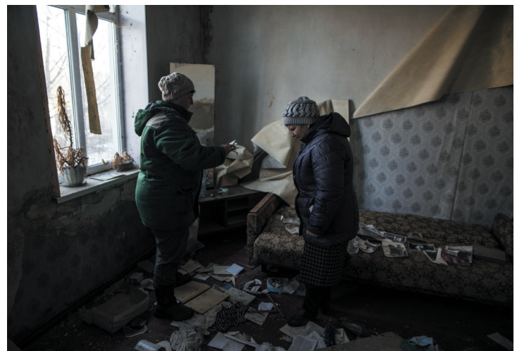
An inspection of the destroyed housing. Photo credit: Ukraine NGO Forum
