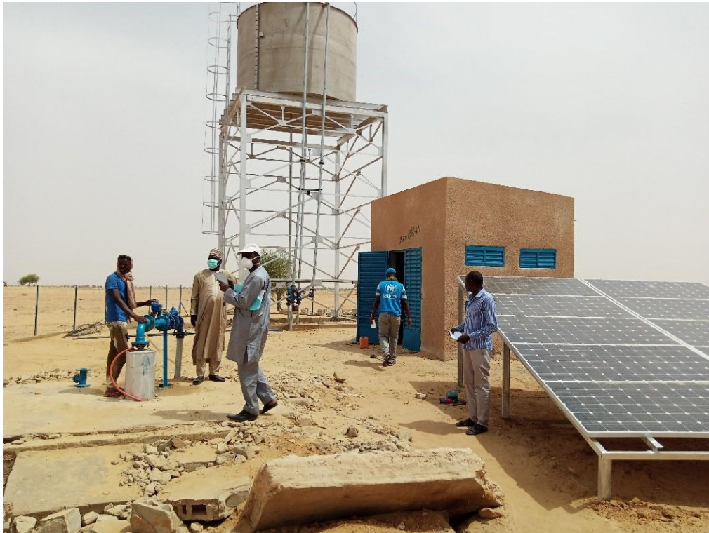
A solar powered well in Assaga, Niger as part of the EU Trust Fund Project on Urbanization in the Diffa region led by UNHCR. ©UNHCR Niger / Médard Monodjomi
