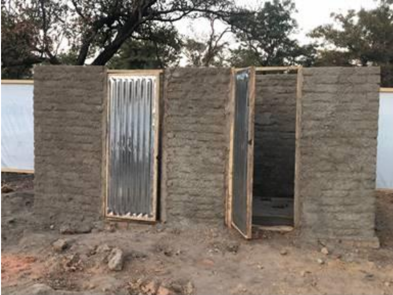
Latrines under construction in Doholo camp ©ADES/ Mbal Innocent
