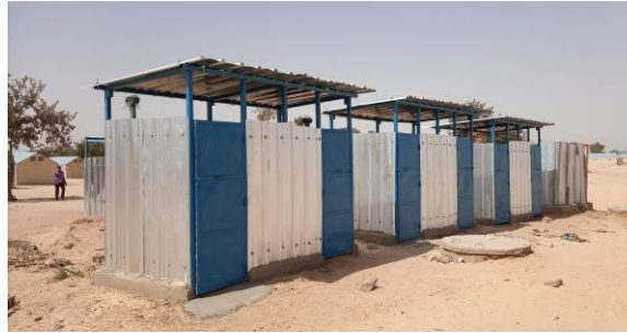
Rehabilitated showers and latrines in Dan Dadji Makaou
