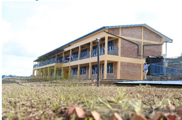
Newly constructed 16 classrooms in Kigeme, Nyamagabe District @UNHCR/Eugene Sibomana
