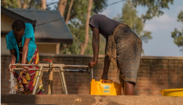
Water distribution point in a refugee camp @Eugene Sibomana
