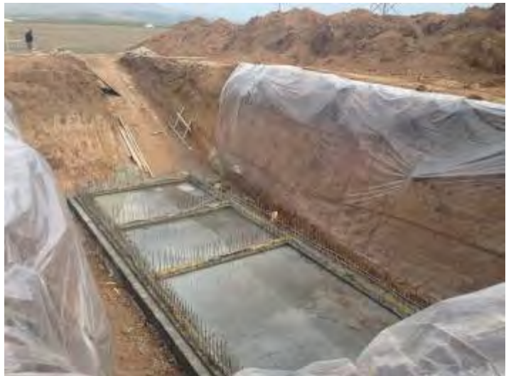
Work on Septic tanks in Arbat camp @UNHCR
