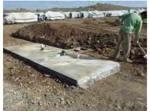
Latrine construction in Kawergosk permanent camp @ UNICEF/C. Muhanika
