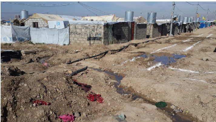
Condition of internal roads and open drainage channel @ UNHCR/S. Gammah
