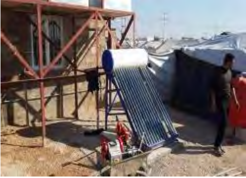
Installing solar heater boilers in the camp@ UNICEF/Majeed
