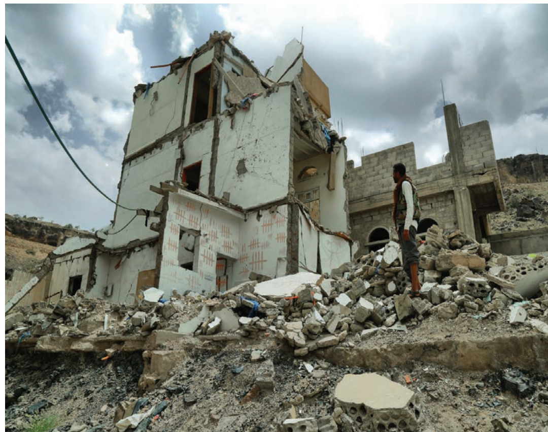
Zakaria Zaki near a destroyed house in Sana'a. He recalls the incident that happened, and the civilians who died after an airstrike targeted the area. Zakaria comments on what he needs by saying "we need the economic situation to get better and this dispute has to stop immediately". Zakaria lives in Sana'a, and has witnessed, and still witnessing many incidents in due to the unsettled conflict. ©UNHCR/Shohdi Alsofi
