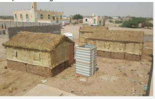
A Transitional Shelter Unit (TSU) is built with iron pipes and local materials. It withstands extreme weather conditions, such as heavy rain, strong wind, humidity and heat. This longer-term shelter solution can last up to five years with proper maintenance
