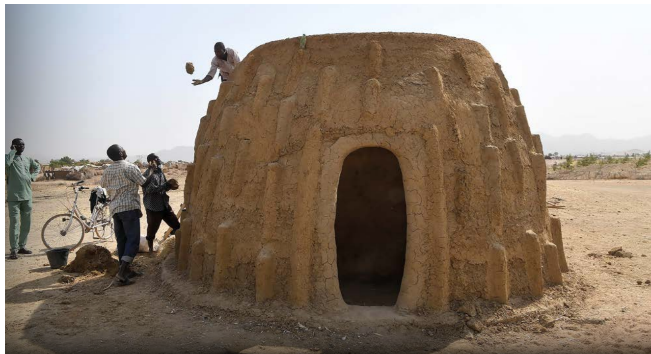
A Nigerian refugee works on the construction of a traditional house made with dried mud in Minawao refugee camp, in Cameroon. This house is a test case and, if successful, could be used more widely to provide sustainable shelters without using wood.
