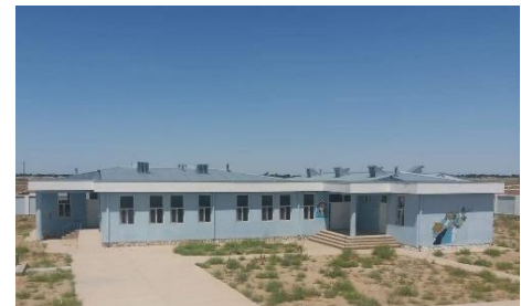
Through its community-based protection programme, UNHCR constructs a secondary school along with a water well. © UNHCR
