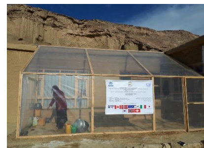
UNHCR provides solarized verandas to returnees to keep their homes warm during the winter months. © UNHCR
