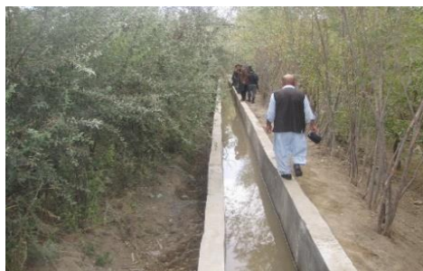
Constructed through cash-for-work initiatives, this water canal supports irrigation to increase farmers' incomes. © UNHCR
