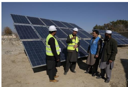
UNHCR supports communities through the development of solar energy projects. © UNHCR/S.Rich
