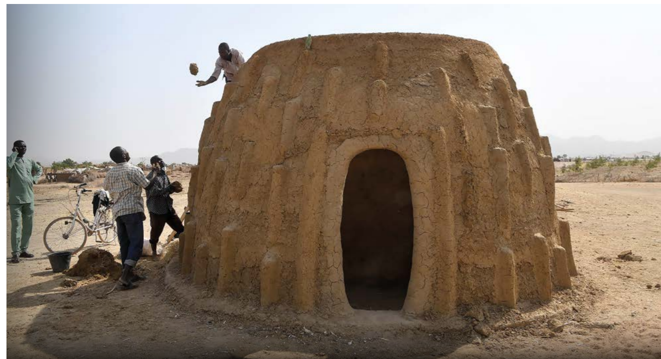
A Nigerian refugee works on the construction of a traditional house made with dried mud in Minawao refugee camp, in Cameroon. This house is a test case and, if successful, could be used more widely to provide sustainable shelters without using wood.
