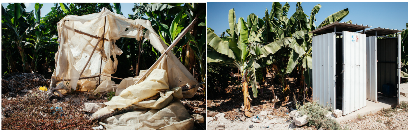
Before and after: A primitive latrine (left) was constructed by refugees in Aaddousiyeh, South Lebanon. It presented significant protection risks, especially for women and girls, as well as environmental and health concerns. In response UNHCR replaced this with three standard latrines (right) connected to a cesspit, providing a significant health and protection improvement for the families concerned. ©UNHCR/Martin Dudek
