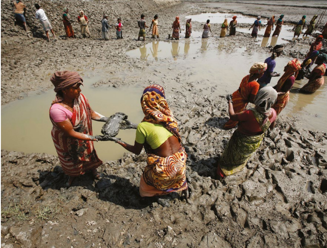
Women work to rebuild an embankment in one of the regions hit by Cyclone Aila in Dacope, Khulna, Bangladesh.
