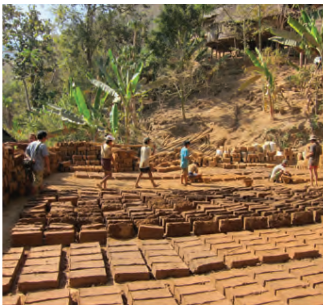
Mudbricks being made to build warehouses
