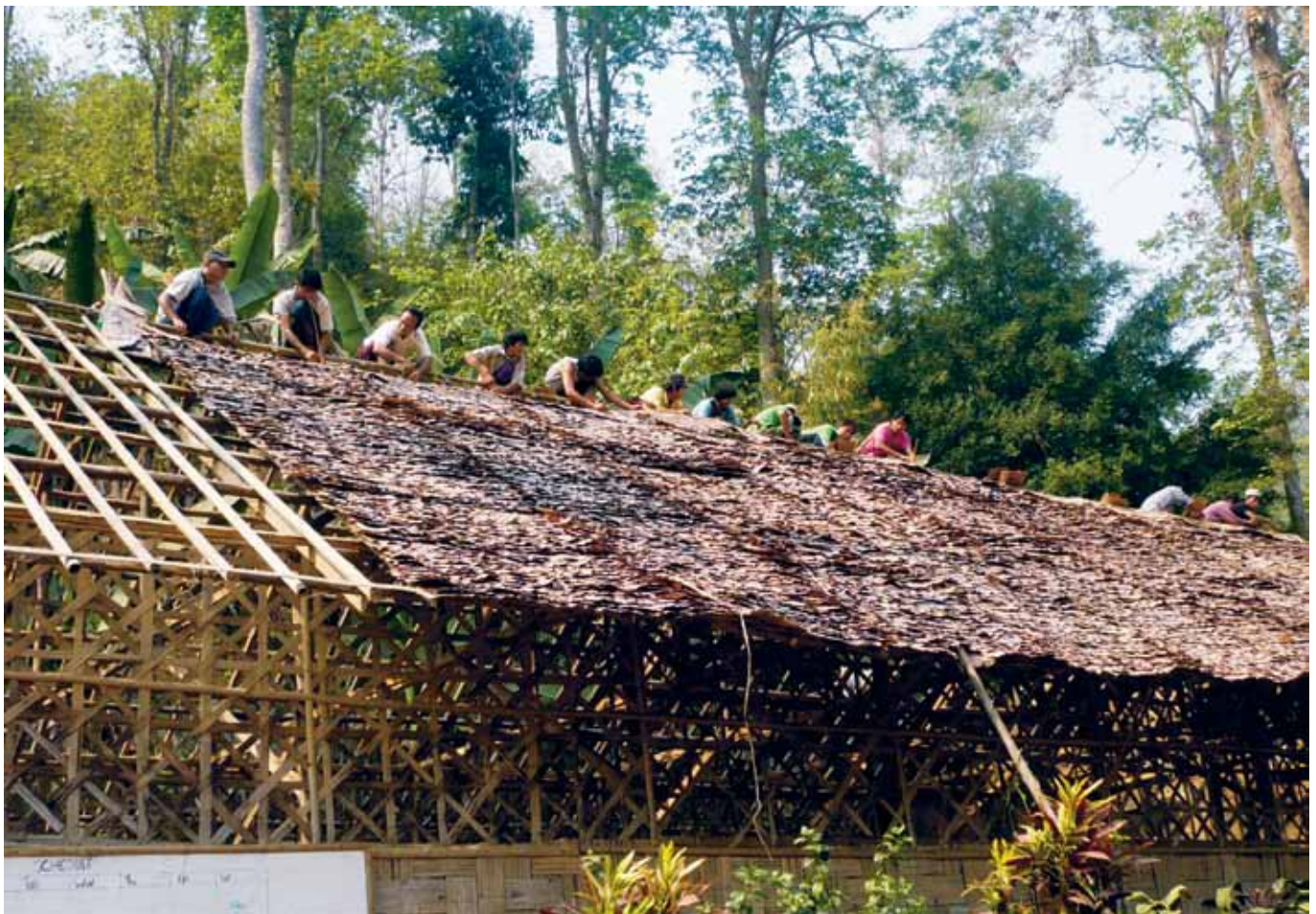
Repairing the roof
