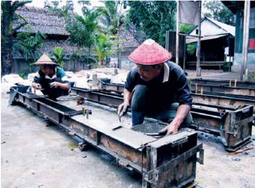
Production of concrete posts, Nu Po
