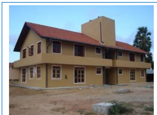
View of Quarters in Mullaitivu DH, Photo Credit: UNOPS©
