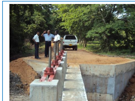
Section of the anicut being constructed in Kokkeliya, Photo credit: IOM©
