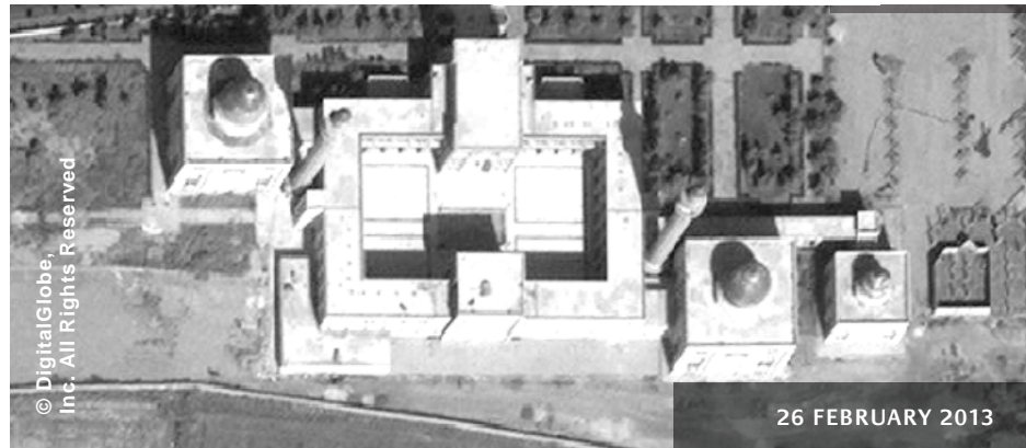
FIGURE 38 Extensive damage to the buildings and structures of the Uwais al-Qarani and Ammar Bin Yasser shrines in Ar Raqqa.
