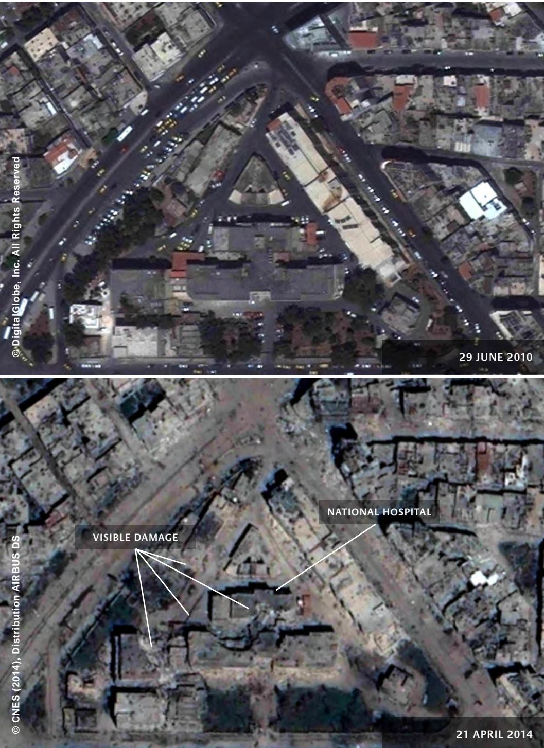
FIGURE 24 Heavy damage at the National Hospital complex in the Jouret Al Shayyah neighborhood of Homs.
