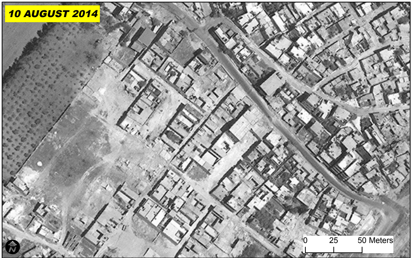
Figure 3: Destroyed structures in Aleppo
