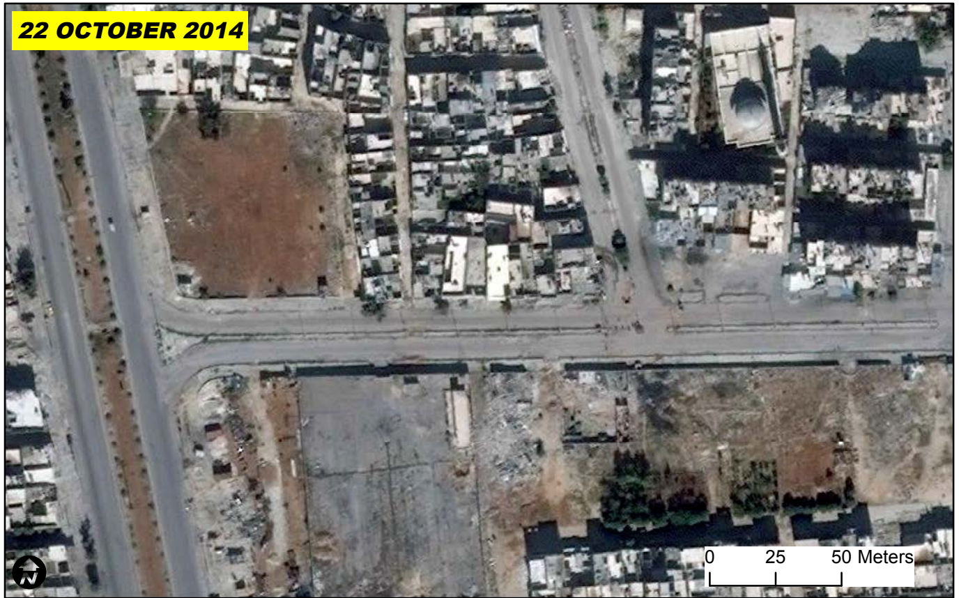
Figure 2: Severely damaged structures in Aleppo
