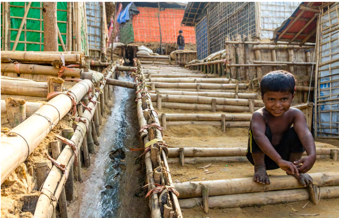
Rafiq, 5, sits on terraced bamboo steps that were part of the community-led settlement improvement activities built through the shelter and markets programming in Zone BB. From left to right, the photo show: Latrine (green), cement-lined bamboo drainage, terraced bamboo steps, vertical bamboo retaining walls and upgraded shelters. Photo by Christopher Reichert for CRS/Caritas Bangladesh.
