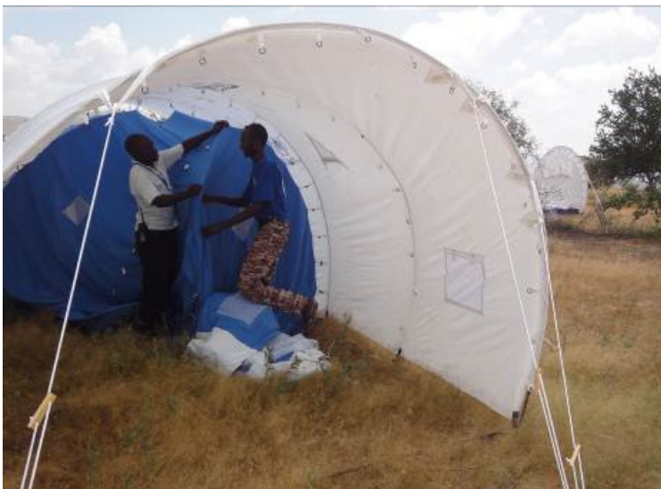
IOM staff erecting a tent in Ifo 2 East Camp
