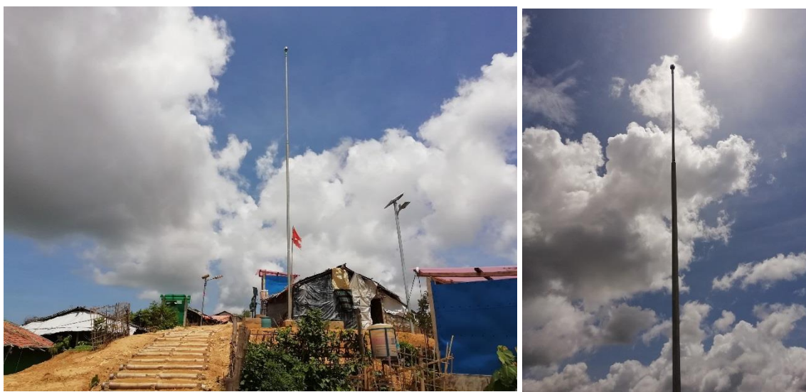
Lightening arrest poles distributed throughout the camp helping to make settlements safer. Photo: UNHCR/S. O'Brien
