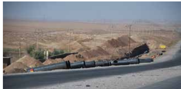
Excavation work in the Right Bank Water project before ISIL © UN-Habitat / Iraqi Urban Observatory
