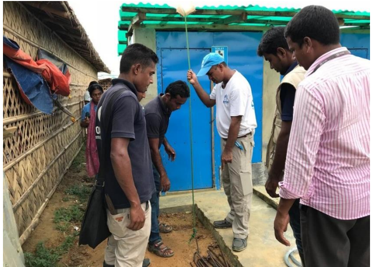
A UNHCR staff shows how to tie down a latrine in preparation for the cyclone season. ©UNHCR/C. Gluck
