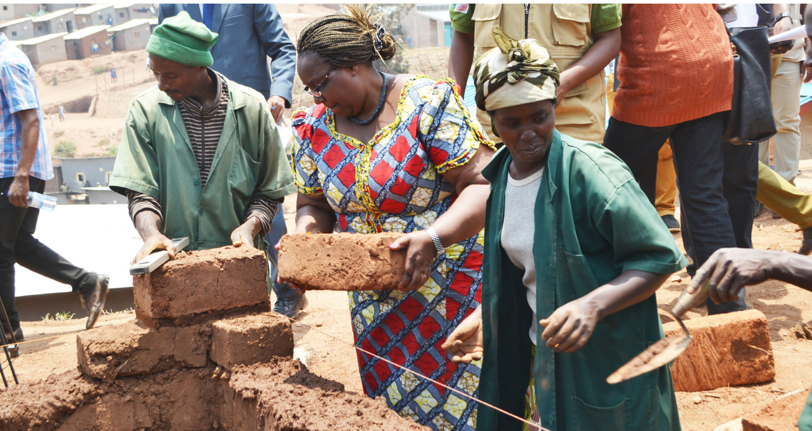
Hon. Seraphine Mukantabana supporting construction efforts in Gihembe camp (2016)
