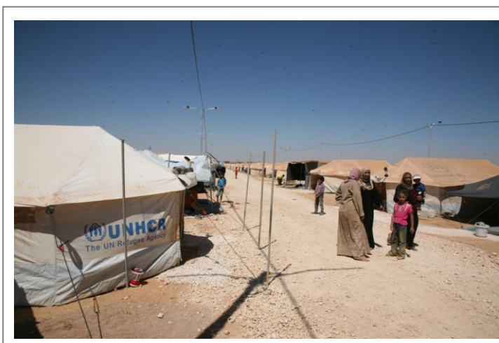
Electricity is being installed at the Za'atri camp ©UNHCR /2012
