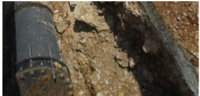
New water distribution pipe in Koura Photo credits - CISP
